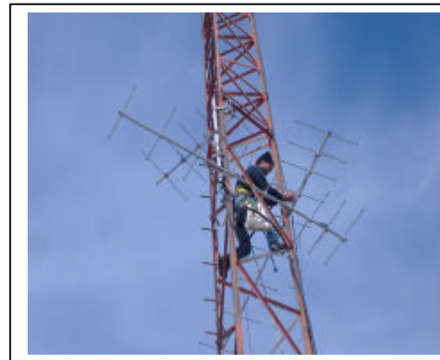
Figure 2. Assembling Yagi directional antennas on one of the towers of the array.
